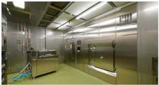
Sterilzation booth, second floor—Three sterilization methods: 1) autoclave, 2) dry-heat sterilizer, and 3) dry-type VHP
