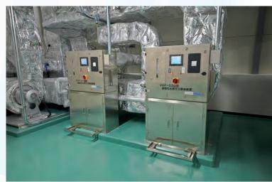
Dry type hydrogen peroxide sterilization system (in machine room, second floor) ) (newly developed in the project)
