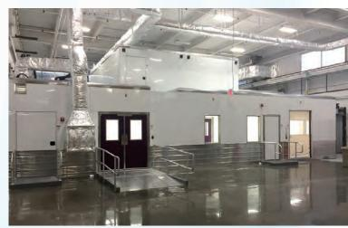
Exterior image—Fully installed PCMM POD in Pfizer facility
